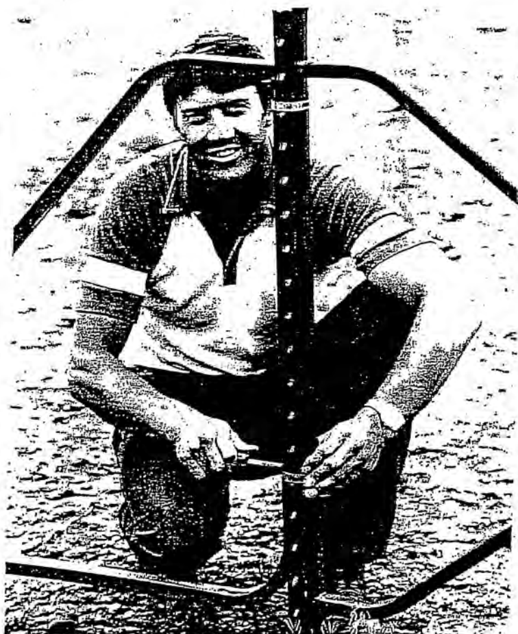
D. For single T-post gate opening double post and clamp together.
